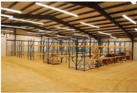
Inside the Warehouse Building
