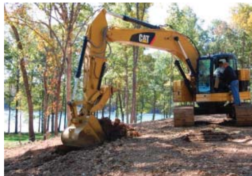
Dr. McKean in the Excavator
