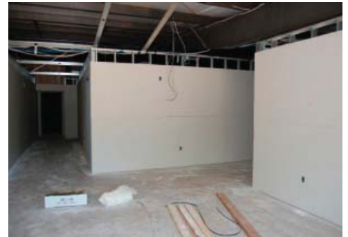
Finished Drywall in the Office Areas
