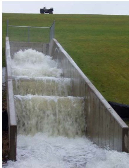
The new spillway generates an awesome sound!
