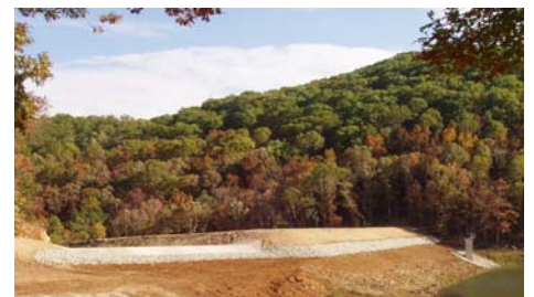
A view of the completed dam shows the intake tower on the far right and the emergency spillway on the left hand side of the picture.
